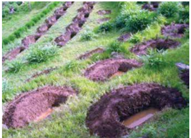
Springshed trenches complemented by vegetative measures were part of Dhara Vikas Programme of RM&DD in Sikkim State.
