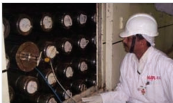
Cutting of Bellow Lip at KAPS
