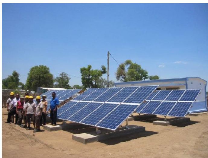
Figure: 10 kilowatt solar plant at Itofaka, Madagascar © credit Fondem
