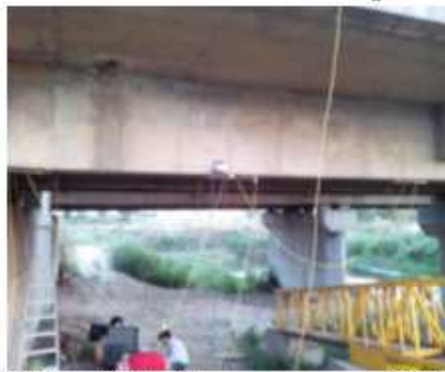
(C) The Bridge Site
