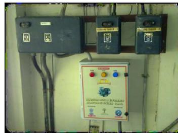
**View of the Power Interfacing Unit fabricated & installed at Site**
