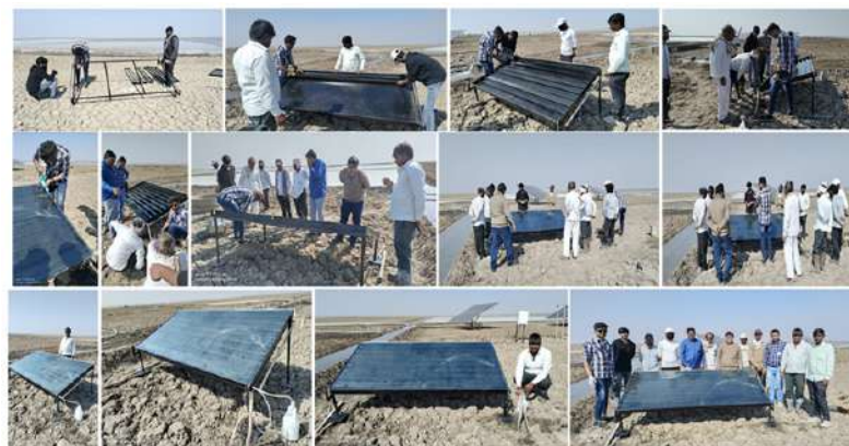
Figure: Installation of solar still unit at Halvad site, CSMCRI Gujarat
