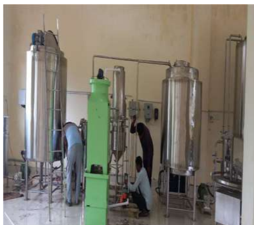
Figure: Honey processing and bottling plant at Karnataka State LAMPS Co-operative Federation building, Mysuru
