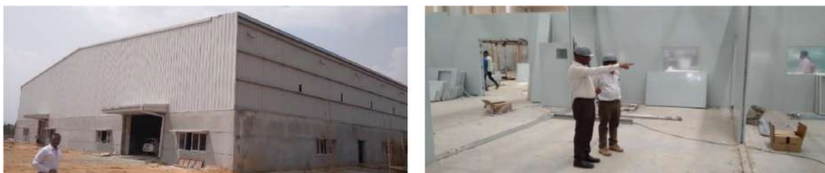
Figure: LIB Pilot facility at Nsure Reliable Power Solutions, Bengaluru
