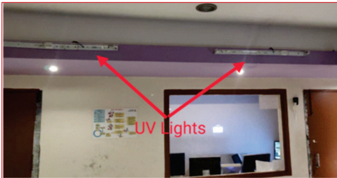
Figure 6: CT room with installed UV lights
