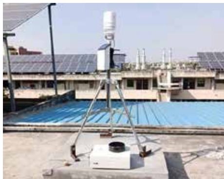
Fig. Installation of custom-designed Automatic Weather Station (AWS) on the top floor of V Block at IIT Delhi, alongside a size comparison with the ATMOS41 weather station.
