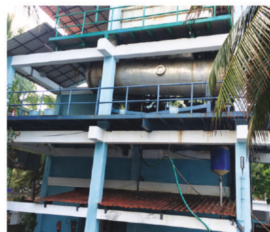
Fig. 2.6: A Close View of LTTD plant at Kavaratti Island
