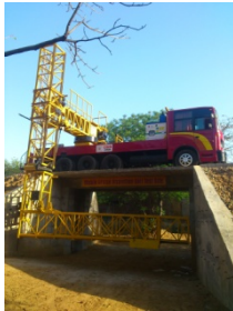
The MBIU under operation on a bridge
