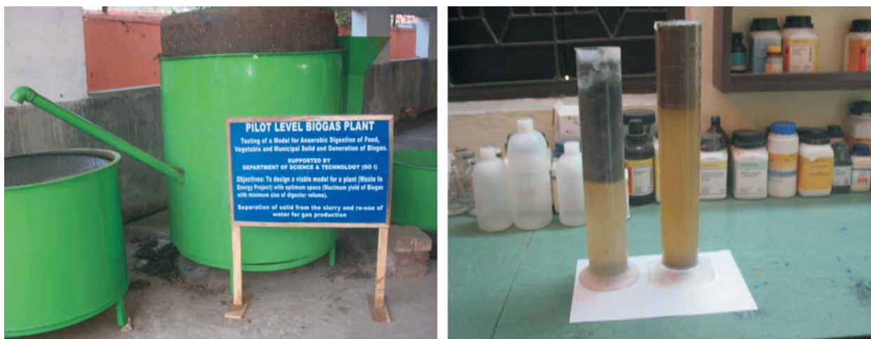
Digester with 1400 L capacity
