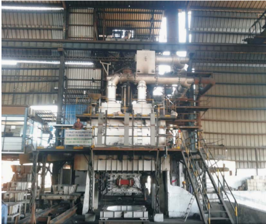
Fig. 4.69: Main CONTIFUR with control room
