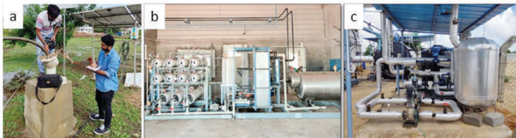
Fig. a) RBF well at Navelim Goa Sal River Site. .b) Forward Osmosis system installed at Narippaiyur Village, Ramanathapuram District, Tamil Nadu. c) Solar hot water system installed at Narippaiyur Village, Ramanathapuram District, Tamil Nadu
